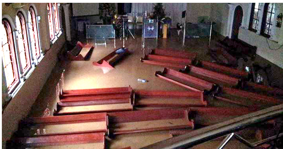
The Paal 2 Adventist church in Manado is submerged in water after days of torrential rains that caused landslides and flooding. (photo provided by Bryan Sumendap)
